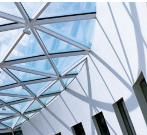
Swinhay – Gloucestershire, UK
