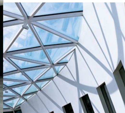
Swinhay – Gloucestershire, UK
